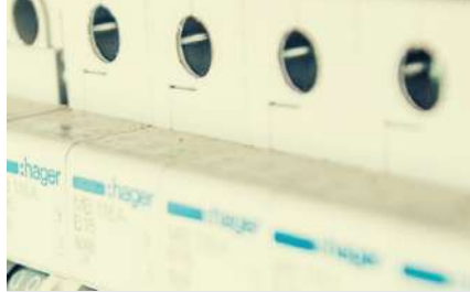
EICR (Fixed Wire Testing)
