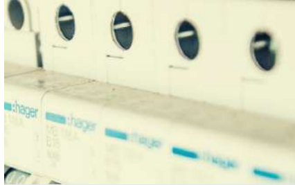
EICR (Fixed Wire Testing)
